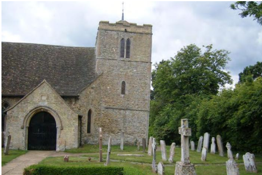
© East Cambridgeshire District Council
